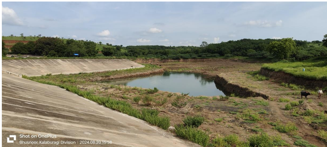
Figure 18: Site image of check dam, which is located at Aland unit premises
