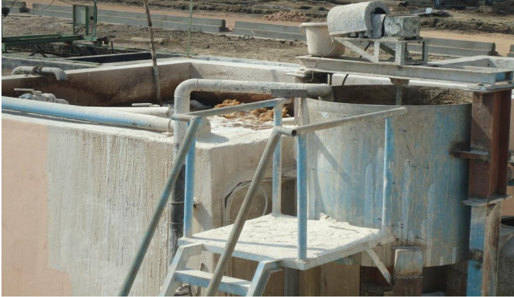
Neutralization Tank
