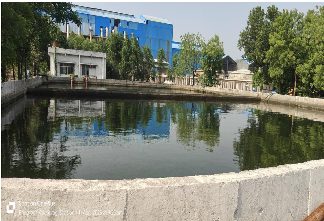
Figure 21: A RCC water tank arranged to collect rooftop rainwater during the rainy season
